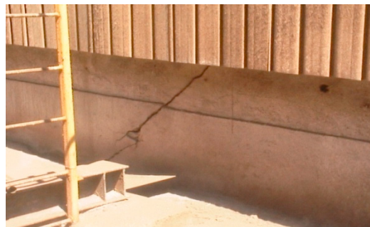
Fig. 4. Cracking 45 degree to both directions and both side of joint.
